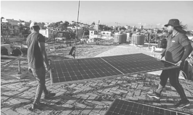
Technicians carry a solar panel on the rooftop of a building in Havana. Cubans face an energy shortage brought on by a recent intensification of the U.S. economic blockade.
