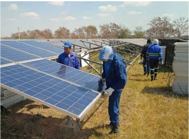
Cubans install solar panels donated by China.
