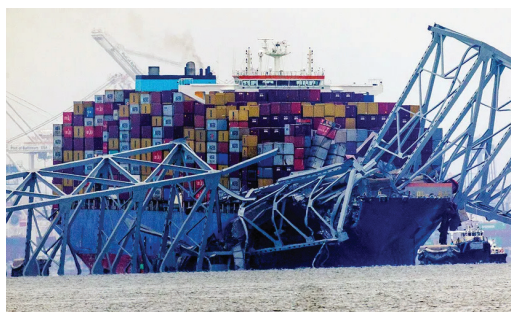
Cargo carrier Dali under portions of collapsed Key Bridge. Baltimore, Maryland, March 29, 2023.
