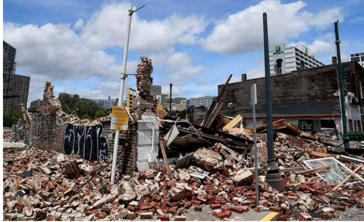
Hurricane Ida damage in Louisiana.
